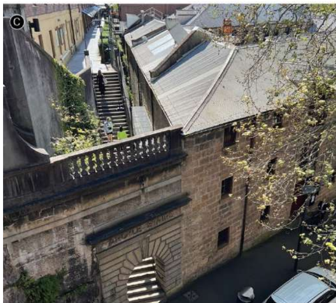
Argyle Stairs can be seen from above from Cumberland Street in the daytime
