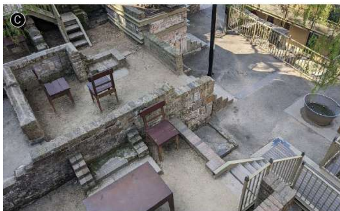
Intricate spaces and interpretative artwork at Foundation Park provide interest, especially in the day time
