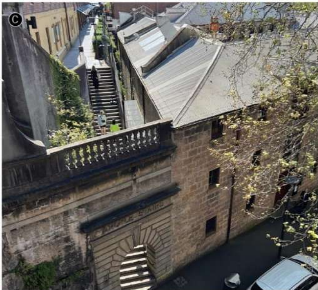
Argyle Stairs can be seen from above from Cumberland Street in the daytime
