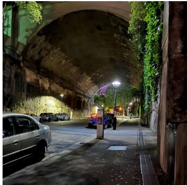
Figure 16: Argyle Cut underpass on Argyle Street
