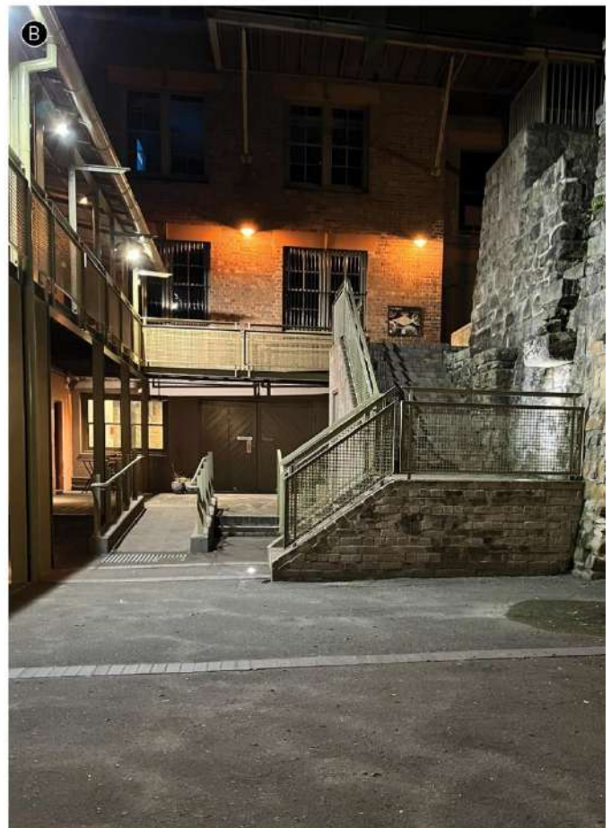
Lower levels of Foundation Park have limited activation and glare lighting at night
