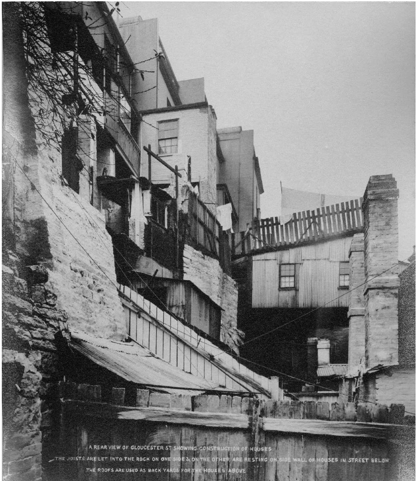
Figure 57: Foundation Park (from the rear of Playfair Terrace), 1901, Bertie Collection, PMNSW Archives
