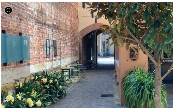
View east down Sargents Arch which connects Nurses Walk to George Street
